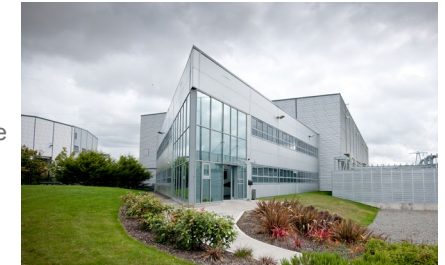
Equinix Dublin IBX data center
